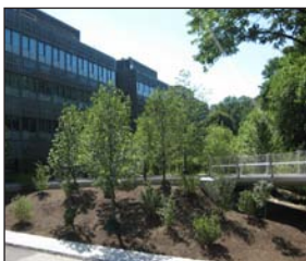
Princeton University Chemistry Building
